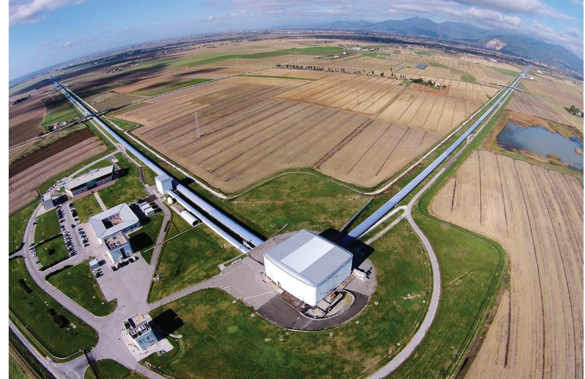
The 1.9-mile-long (3 km) arms of the Virgo interferometer are nestled in the countryside near Pisa, Italy. This instrument works in tandem with the twin LIGO interferometers in the United States.
